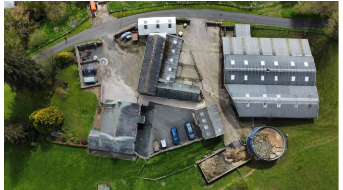
Aerial View from North
