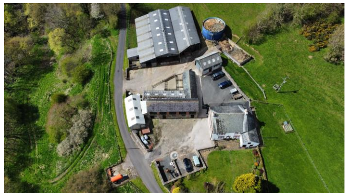
Aerial view from South East
